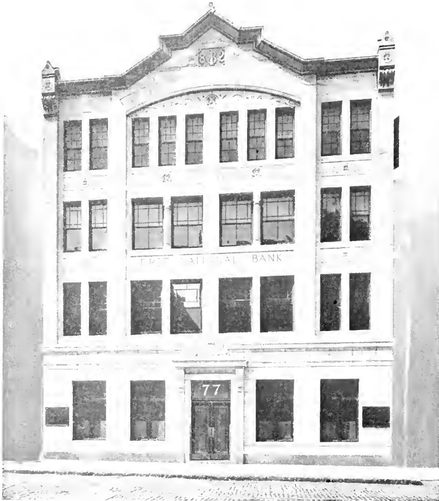
FIRST NATIONAL BANK BUILDING, 73-79 WASHINGTON STREET
